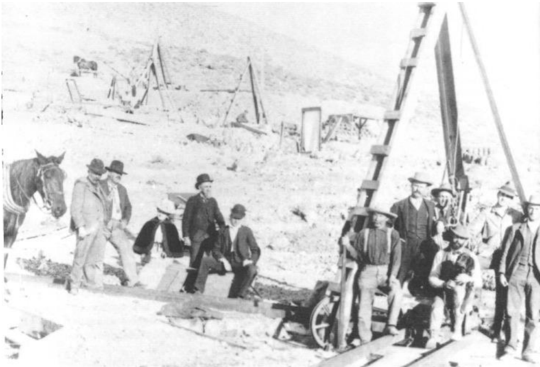
In 1901 leases were being worked and were more developed with small headframes built over the shafts. Ore was hoisted out of the shafts by means of a whim that was powered by the horse at the left. From left are Cal Brougner, Jim Butler, Belle Butler, E.W. Smith, who took the photograph, a group of leasers, and Tasker Oddie at the far right. Central Nevada Historical Society — Ira Jacobsen Collection
