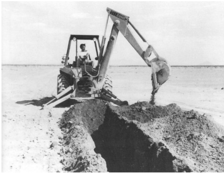
Digging a ditch to install a 10-inch water line to supply a sprinkler system in the Amargosa Valley (circa 1980). Nye County Town History Project—Records Collection
