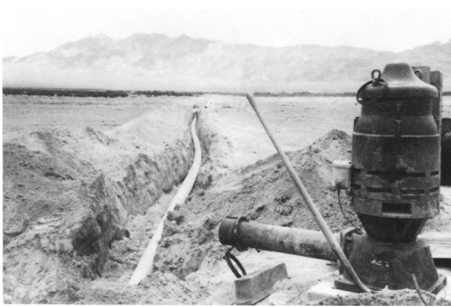
The development of the Amargosa Valley was advanced by projects such as this installation of a 10-inch water line and pump to supply a circle sprinkler system. The 75-horsepower electric turbine pump supports two sprinkler systems with a total of 1,450 gallons per minute. At that capacity, the pump only draws water down 3 inches in the well. Looking southwest toward the Funeral Mountains (circa 1980). Nye County Town History Project—Records Collection
